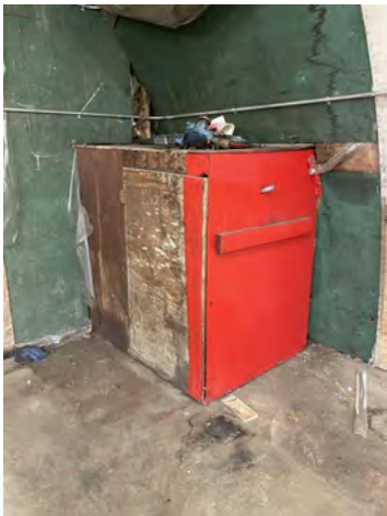
Heat box for former water system. Is located in corner of shop.
