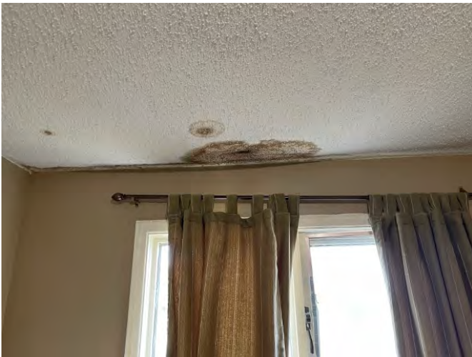
Second of 3 bedrooms in the basement level. This room is under the main (upper) floor bedroom that has water damage. This room also has water damage.
