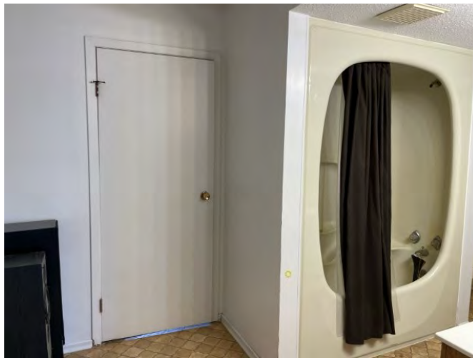
Door in this bathroom provides access to the mechanical room for the home and the pool.
