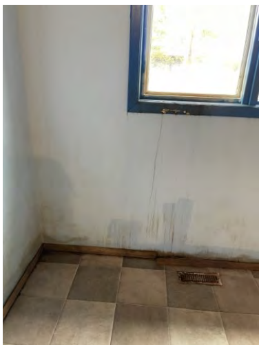
Water damage on wall and ceiling of this bedroom on main(upper) floor.
